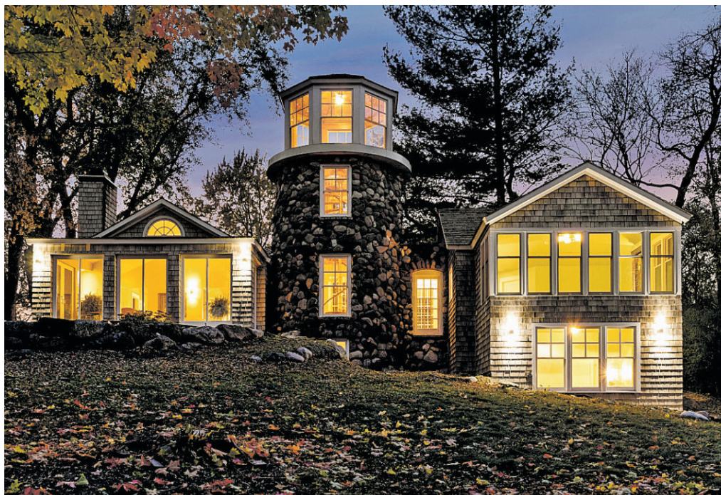
The "Lighthouse Keeper's Cottage" is made up of two cottages that the architect/owner purchased and adjoined with a lighthouse structure.
